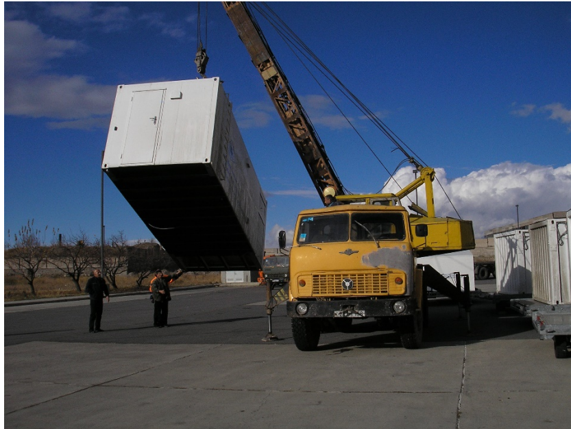
Figure 2. The control room and dome-containers of the module EOP-1 at the airport Zvartnots
