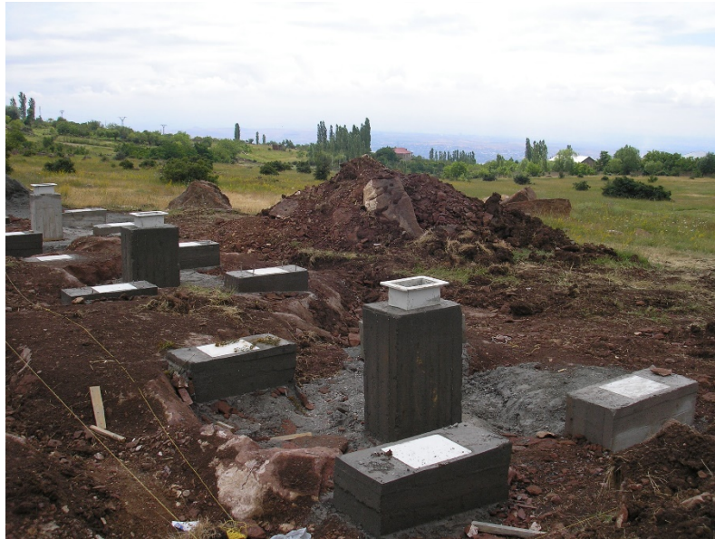
Figure 3. The fundamentals of telescopes and containers-domes built at Saravand.
